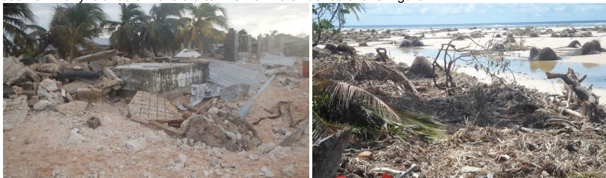
Figure 4 Erosion and damage caused by waves from TC Pam on Nui; and Sand and palm trees scattered across reef to edge following TC Pam on Nanumanga Tuvalu (Source PWD GoT).
