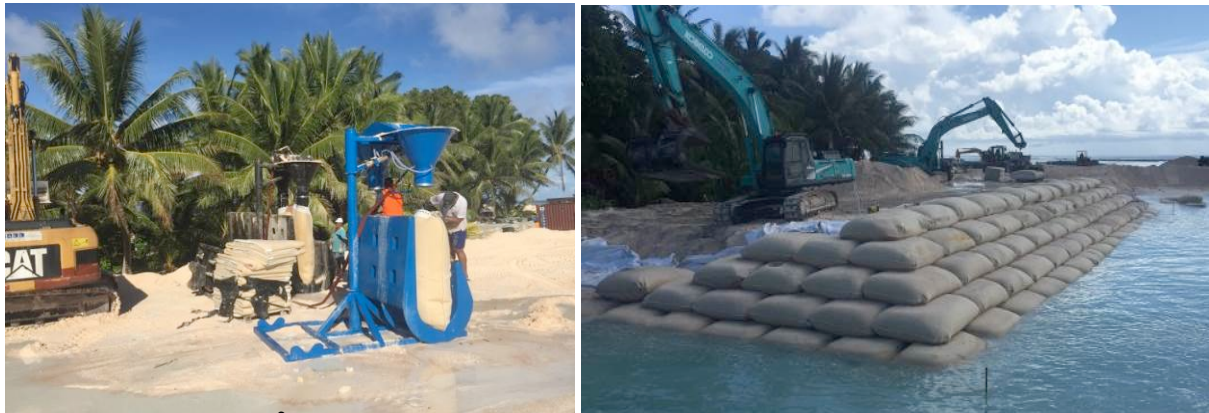
Figure 7 Filling 2.5 m 3 (~4 T) Geobags in a special frame and placing in a seawall - Nukufetau, Tuvalu. Note special attachment on excavator.
