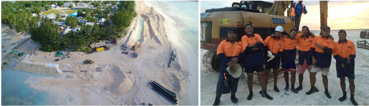
Figure 9 Works in progress and the local construction team on Nukufetau.
