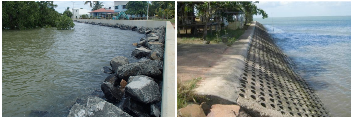
Figure 6 Hard seawalls with rock armour seawall with concrete barrier to exclude high water levels on Saibai, and a rigid seawall of small pattern placed Seabee armour units on Boigu, Torres Strait.
