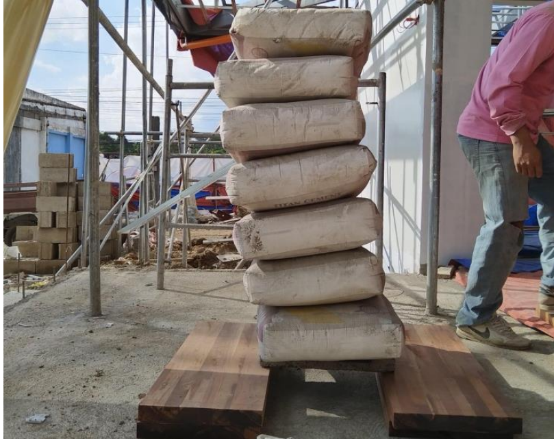
Figure 13. Site Load test.
