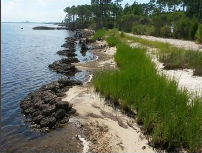
Nearshore: Coastal reefs for wave protection
