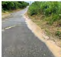
Figure 6: Dirty stormwater runoff being discharged into Capomare Bay.
